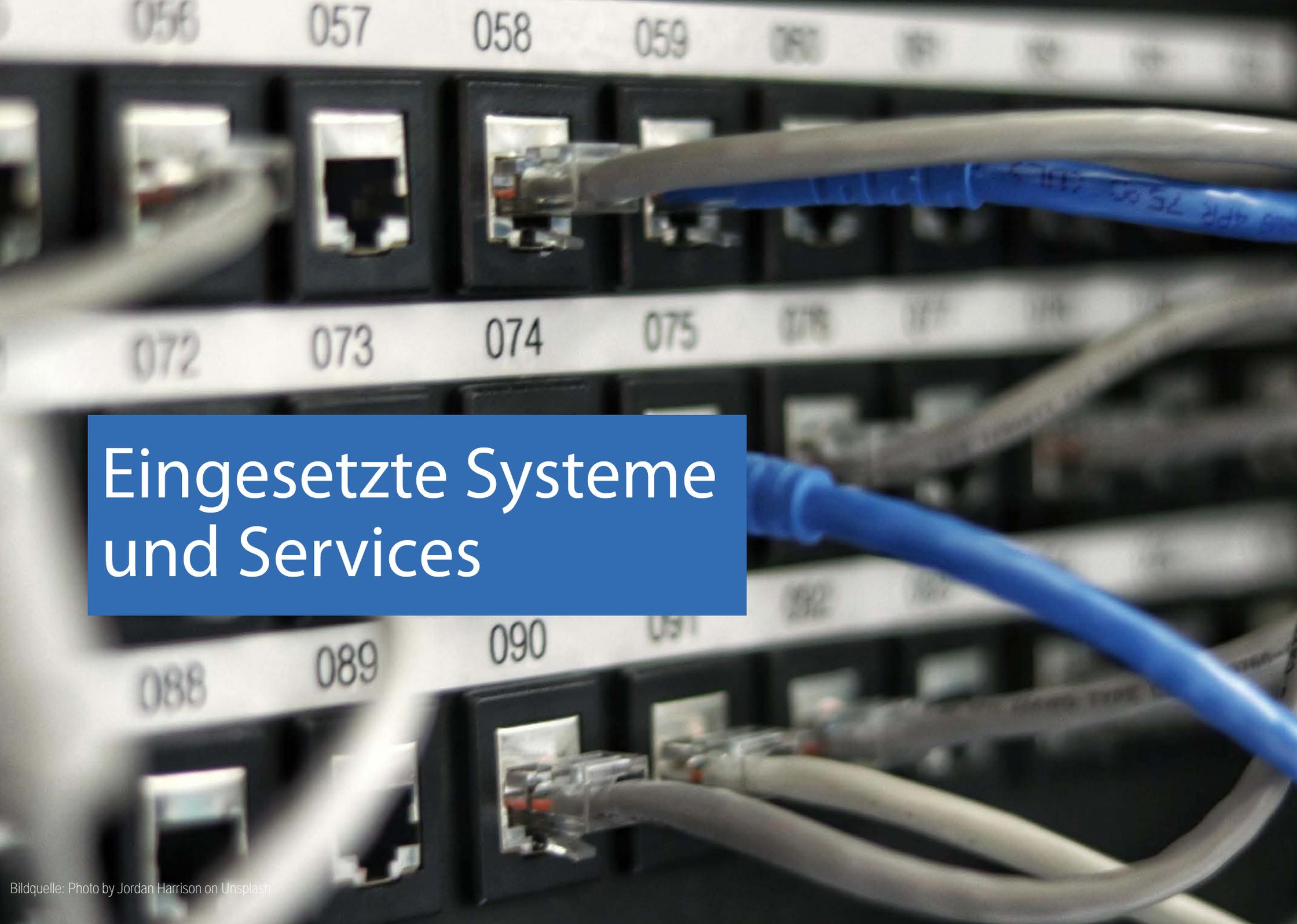
A close-up photograph of a network switch panel. The panel features several rows of RJ45 ports, each labeled with a number. The top row shows ports 056, 057, 058, and 059. The middle row shows ports 072, 073, 074, and 075. The bottom row shows ports 088, 089, and 090. Several grey Ethernet cables are plugged into the ports. A prominent blue Ethernet cable is plugged into port 074. The background is slightly blurred, showing more of the switch panel and other cables.
