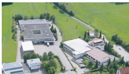
Firmenzentrale METZ CONNECT, Blumberg
