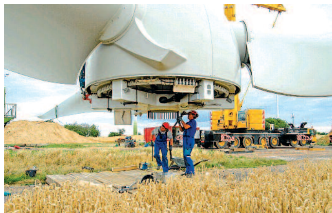
Rotormontage in Nieder-Olm
